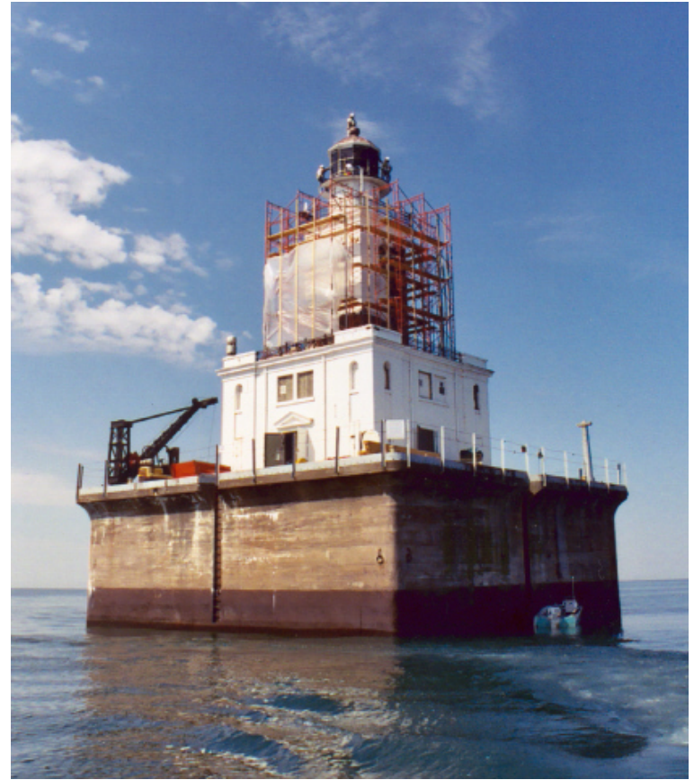
Being restored in 2003
