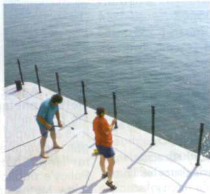
Powerwashing the deck.
