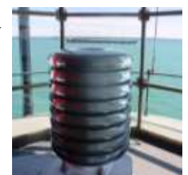
Eight tier VLB-44 in DeTour Reef Light lantern. Laker Paul R. Tregurtha in background (1013.5 feet in length)
