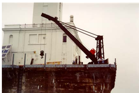
The lighthouse new deck crane completed in 2001 included some original deck crane pieces recovered from underwater by Mike Spears and his dive team.
