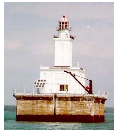
DeTour Reef Light with the newly restored deck crane. Note solar panels on left.
