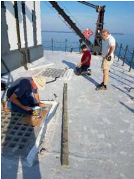
Brian, Ron and Dave working on the sealing the deck lights.
