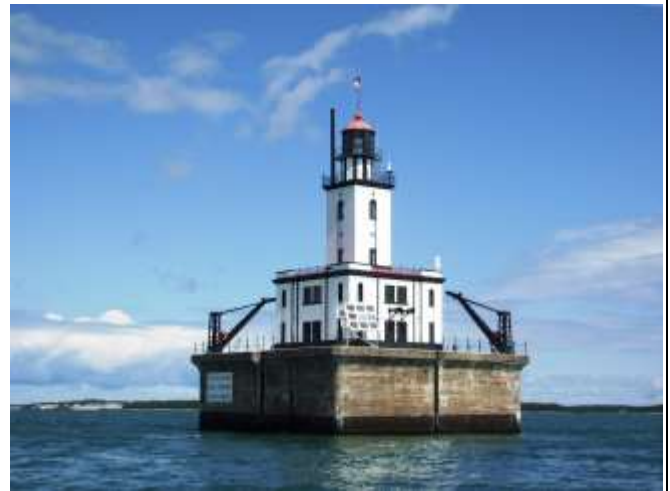
The deck of the DeTour Reef Light will be upgraded this summer with the help of a grant from the Michigan Lighthouse Assistance Program, which is funded by sale of lighthouse license plates. The lighthouse is owned and maintained by the DeTour Reef Light Preservation Society (Photograph courtesy of DeTour Reef Light Preservation Society).
