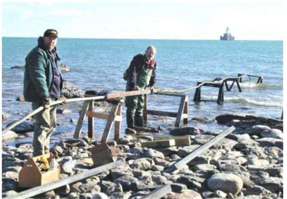
Placing new steel protection on power cable to DeTour Reef Light
