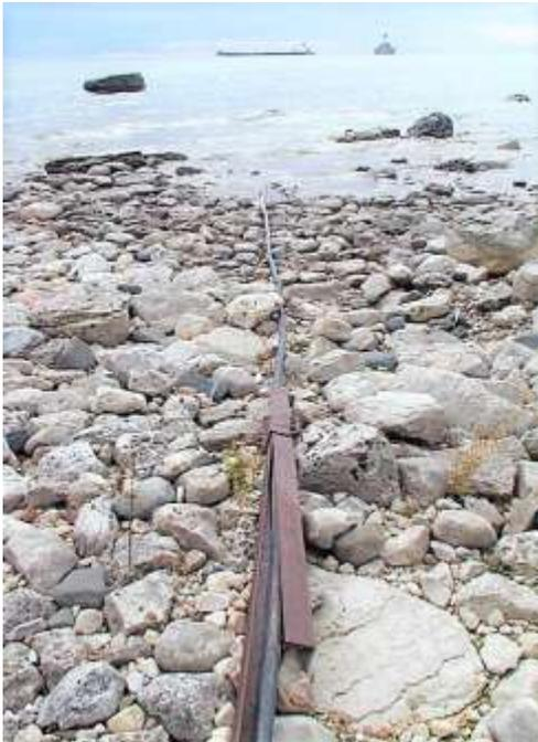
Power cable before 2003 repair to steel protection
