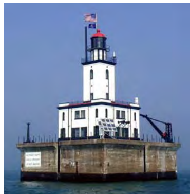
Flags are flying at the newly restored DeTour Reef Light.
