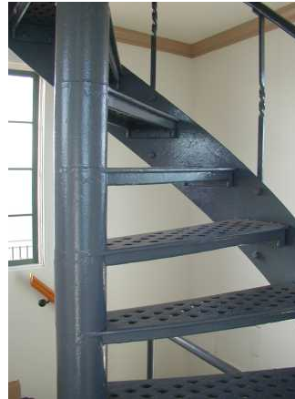
Steps after restoration
