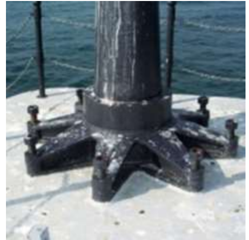
Before the lighthouse Keepers found a solution, cleaning bird droppings was a regular and time-consuming chore.
