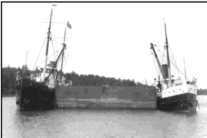
DeTour Reef Light Station crib being towed to offshore site 1930. Photo courtesy of Don Nelson
