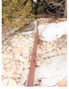
DeTour Reef Light power cable with steel protection looking East toward power pole
