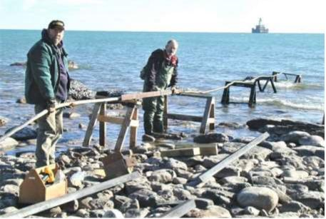
Placing new steel protection on power cable to DeTour Reef Light
