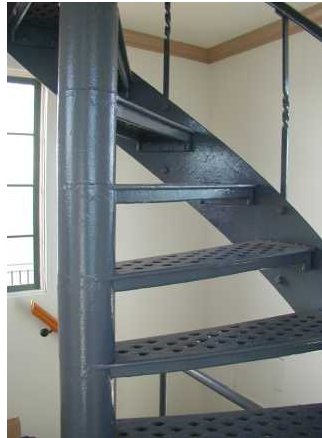
Steps after restoration
