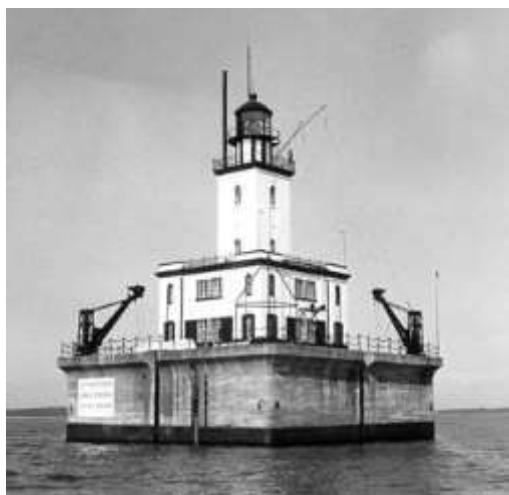
DeTour Reef Light Station 1931
