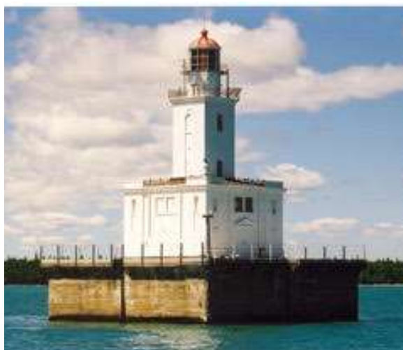
DeTour Reef Light Station 1997 before restoration
