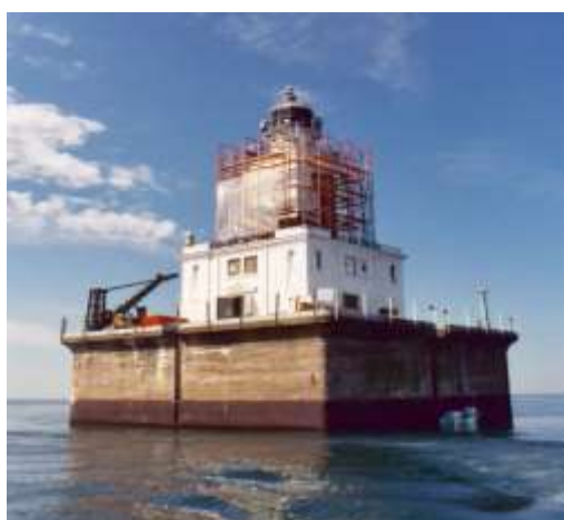
DeTour Reef Light Station Restoration 2004
